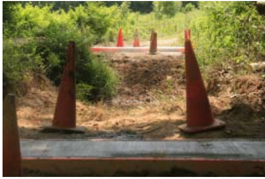
Concrete footings waiting for the bridge
